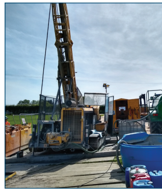
A drill rig set up on a bog mat
